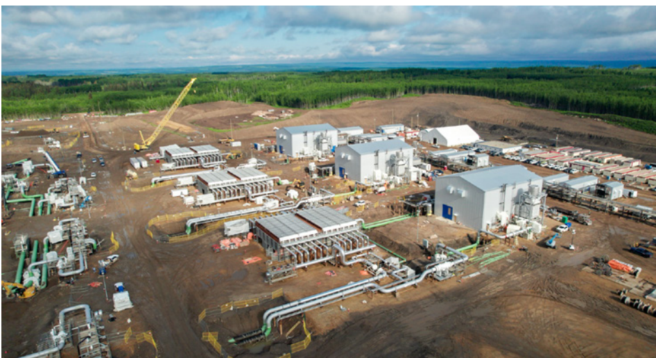
Aerial photo of the Wilde Lake Compressor Station
