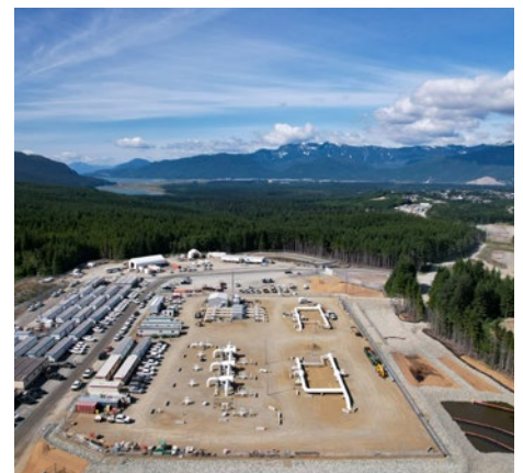
Aerial view of the Kitimat Meter Station.
