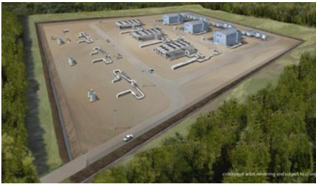
A rendering of a compressor station with three compressor units.
