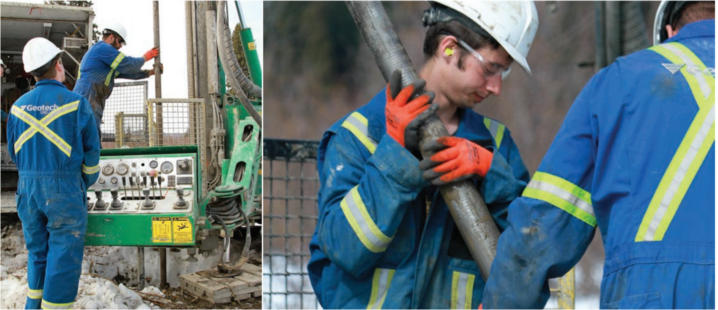
Geotechnical investigation – drilling bore hole
