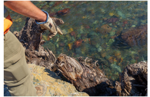
Using root wads from tree stumps provides flow refuge for smaller fish which may not have been available to them before.
