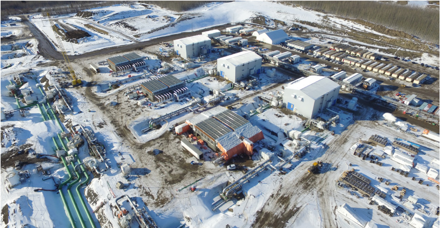
Aerial View of the Wilde Lake Compressor and Meter Station
