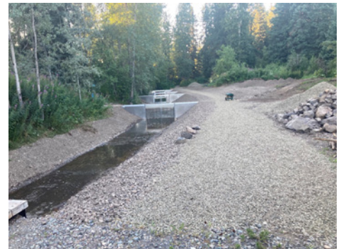
Updated metal barriers at the Toboggan Creek Hatchery
