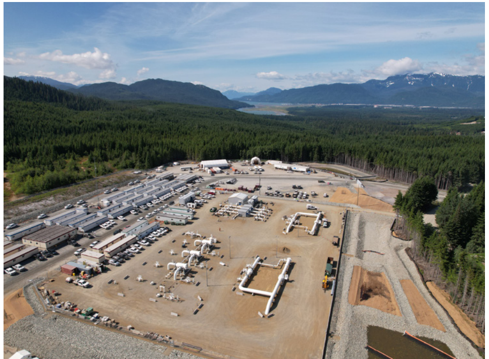
Aerial view of Kitimat Meter Station
