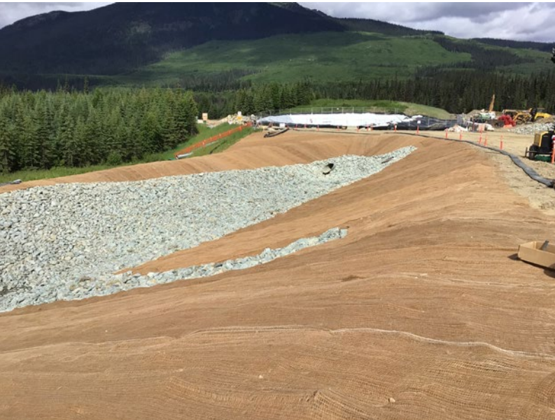
Slope lined with erosion blanket to reduce soil loss, enhance vegetative growth, and improve long-term slope stability.
