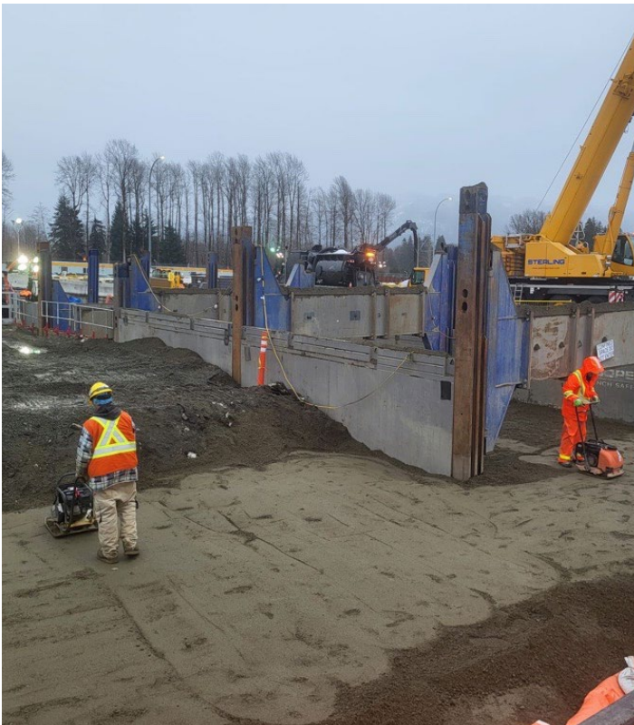
Backfill and compaction of the LNG Link Meter Station NPS 48 piping.
