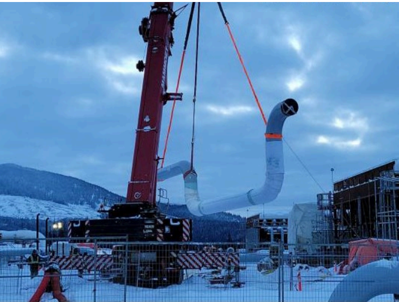
A large bore piping spool being positioned in place ahead of welding.
