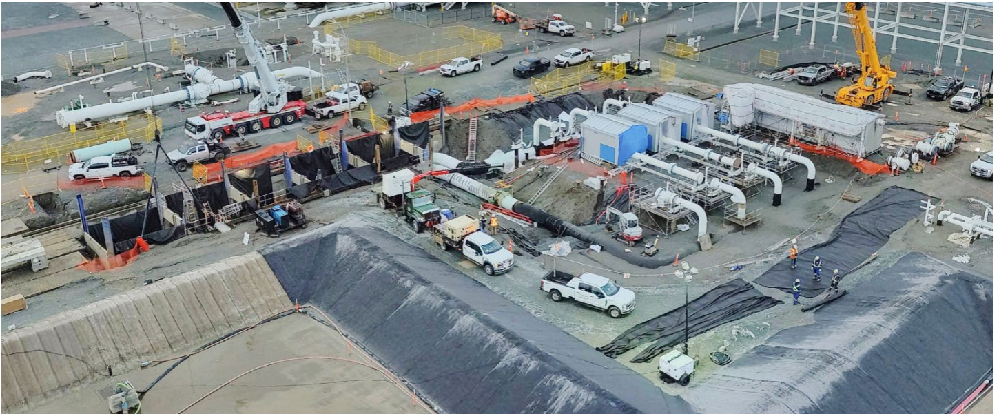
Aerial view of NPS 48 pipe installation around the meter run buildings and NPS 24 headers at LNG Link Meter Station.
