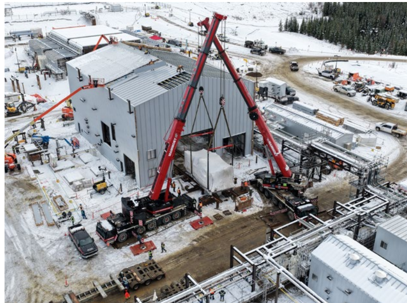
Installation of a turbo compressor in one of the Project's compressor buildings.
