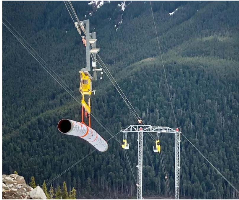
The first segment of pipe being transported up the hill to commence mainline construction
