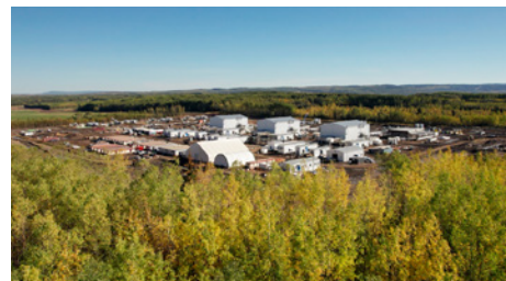
The Wilde Lake Compressor Station serves as the starting point for the 670-kilometre natural gas pipeline in eastern British Columbia and is similar to the five new compressor facilities that will be constructed as part of Phase 2.
