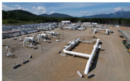
The Kitimat Meter Station, where natural gas is measured and then delivered to the LNG Canada facility.
