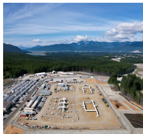
Aerial view of the Kitimat Meter Station.
