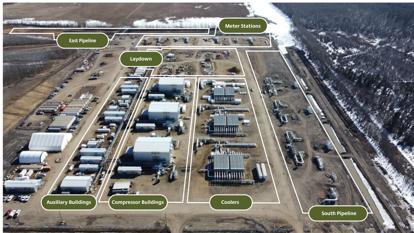
Aerial view of the Wilde Lake Compressor Station.
