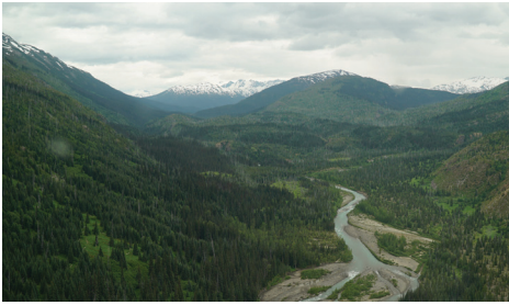
Section 7 of the project, near Houson, B.C.
